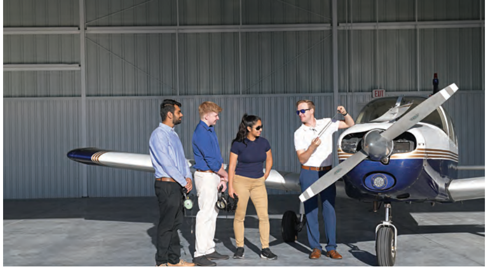
A new hangar at the Schenectady County Airport was unveiled and houses planes and educational space for the College’s Aviation Science program. See more on page 6.
